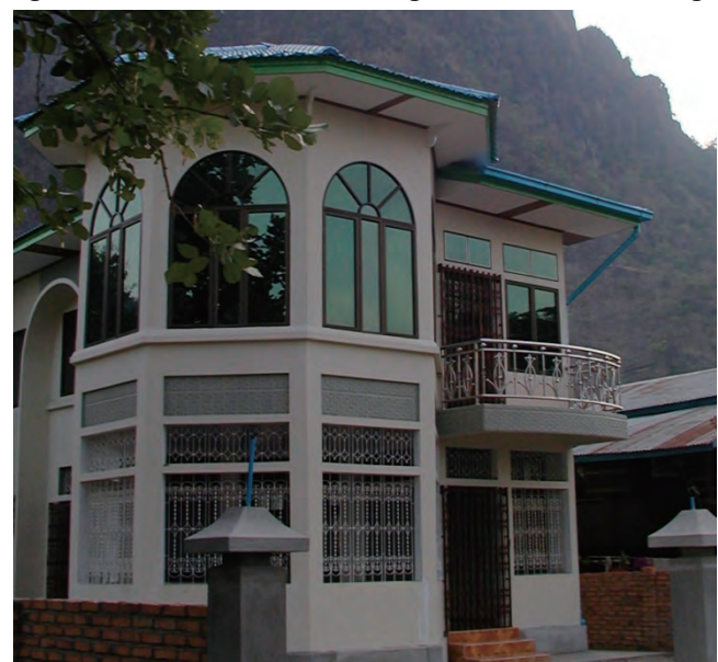
Fig. 2 A migrant-laborer’s house under construction
